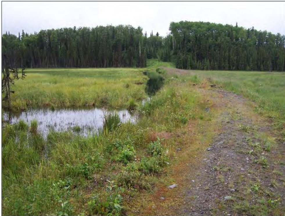
Figure 5. Existing road bed/beaver dam barrier at the outlet of Derks Lake, 2010.
