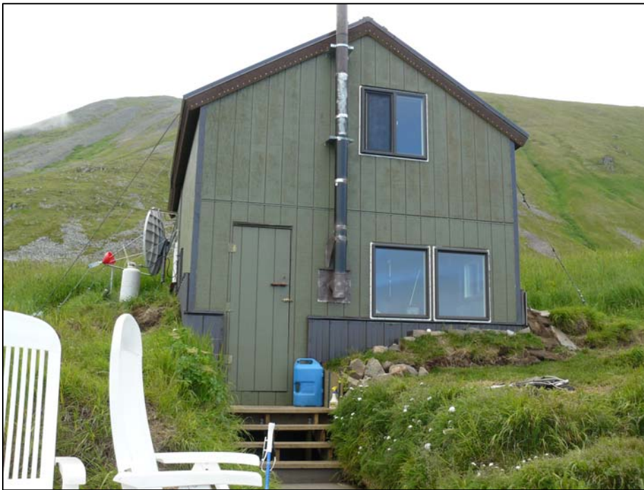
Figure 6. Finished rebuilt Round Island cabin.
